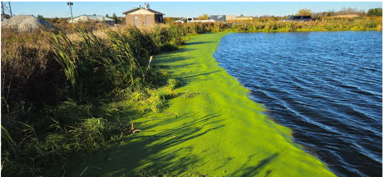
Image. OCWA – Warton Biosolids Aerated Cell 1.
