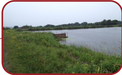
Elm Street Sewage Pumping Station (SPS)
